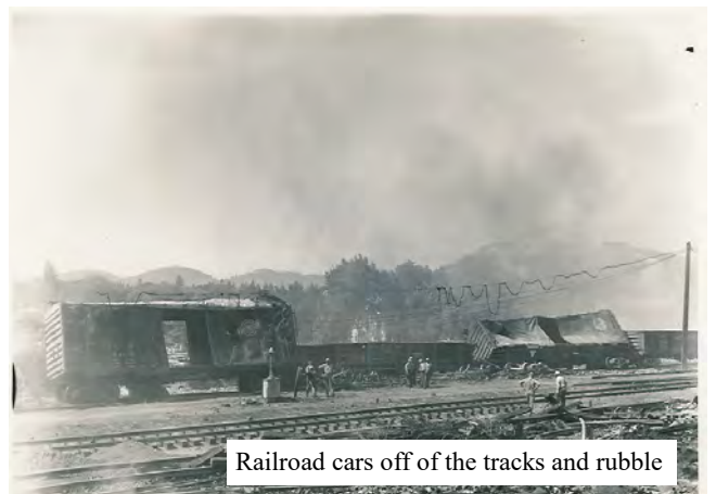
Blast damage in railroad yard
